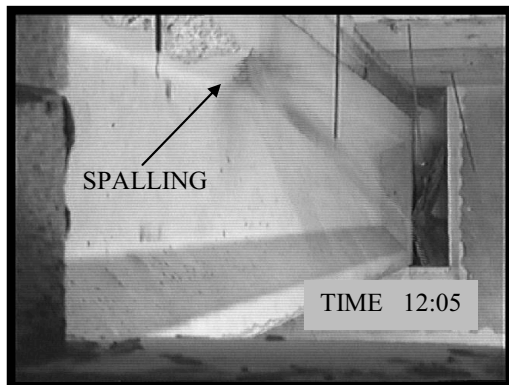
Figure 2.38 Loaded pre-stressed beam tested during the I-beam tests with ISO 834:1977 fire exposure. Spalling starts in the upper flange after 12 minutes of standard fire exposure.
