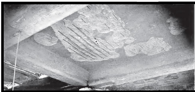
Figure 2.8 Spalling of the concrete cover during a moderate fire after the San Francisco earthquake.
