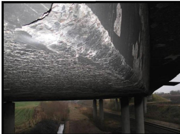
Figure 2.26 Fire spalling from a fire under a bridge. The heat source was solvents burning under the bridge coming from a lorry on the bridge. Photo Lars Boström.
