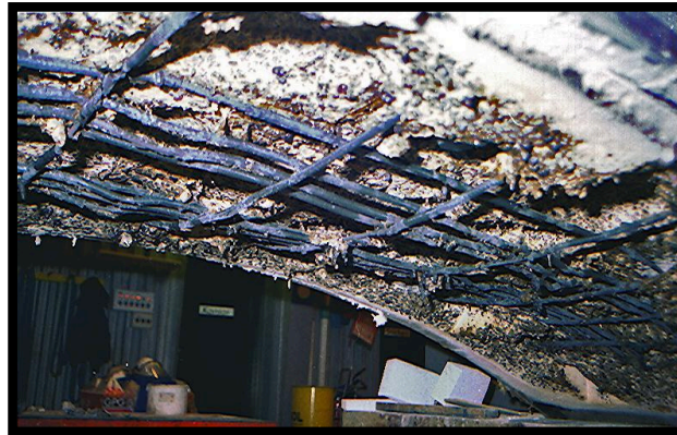
Figure 2.19 Tunnel element from the Great Belt tunnel fire tested at SP Technical Research Institute of Sweden. Photo included in the official report from Trafikministeriet (1995).
