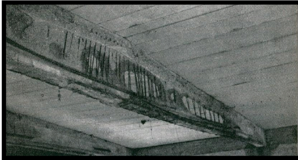
Figure 2.4 Spalling of pre-stressed beams due to fast cooling by adding water described by the Swedish Tariff Association (1959).
